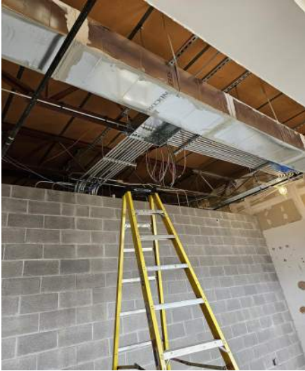
Pulling wire at serving line area
