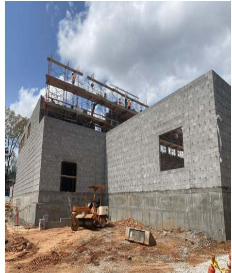
CMU Exterior Walls being installed
