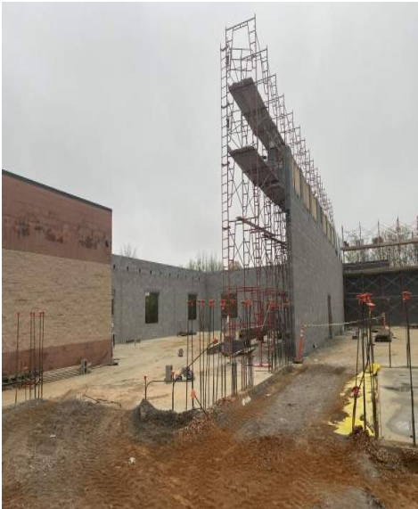
CMU Load Bearing Wall being installed
